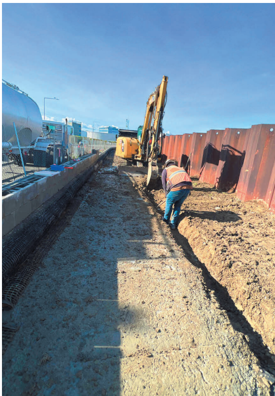
Levee retaining wall under construction
